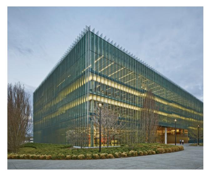
The sloping floor is legible from the completely glazed exterior, whose fritted, 2-foc serve as an external shading device and transfer wind loads.
